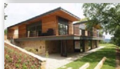
Vila Bystrc, Brno
